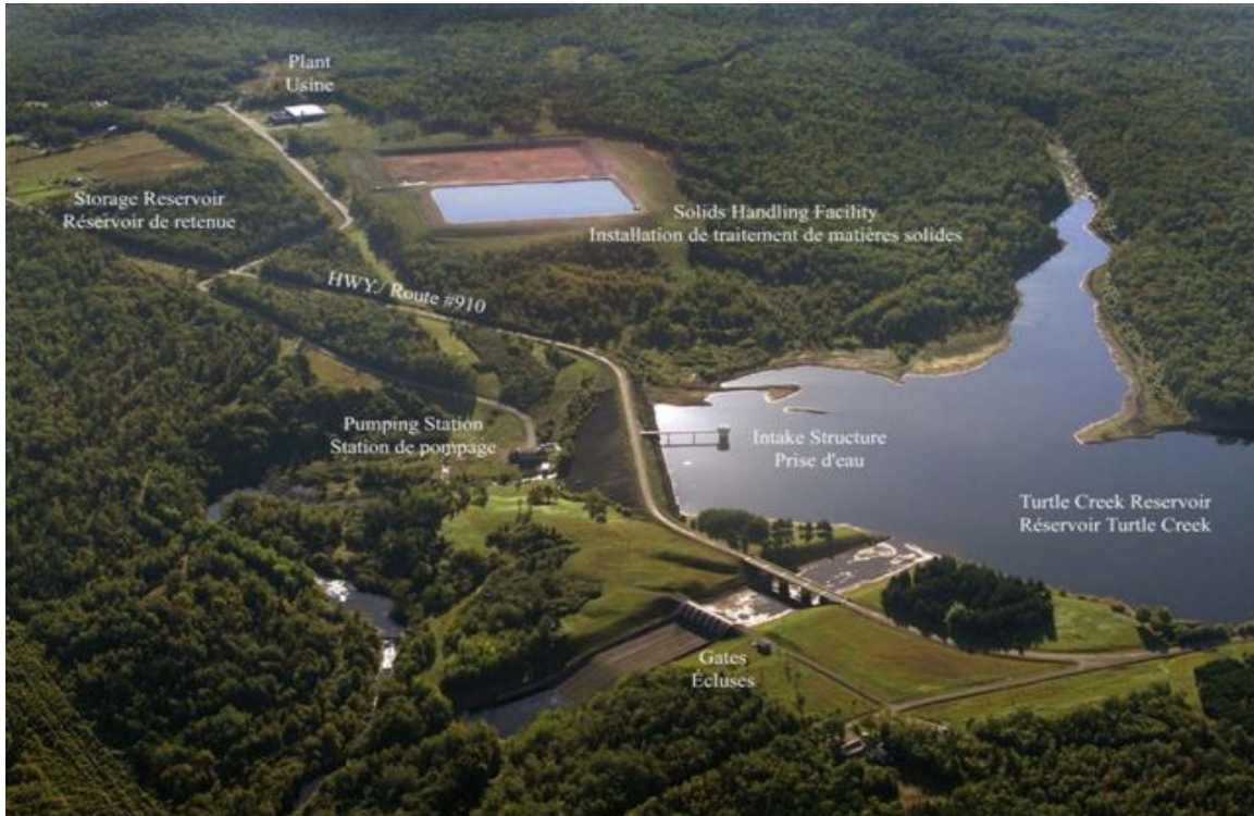
Figure 3.1 Turtle Creek Reservoir and Water Treatment Facility
